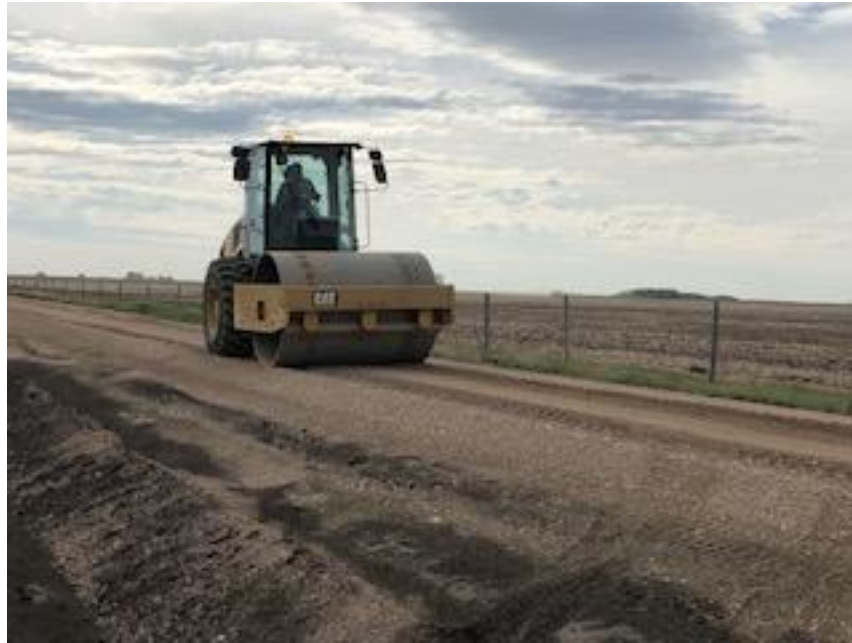
Packer compacting access road
