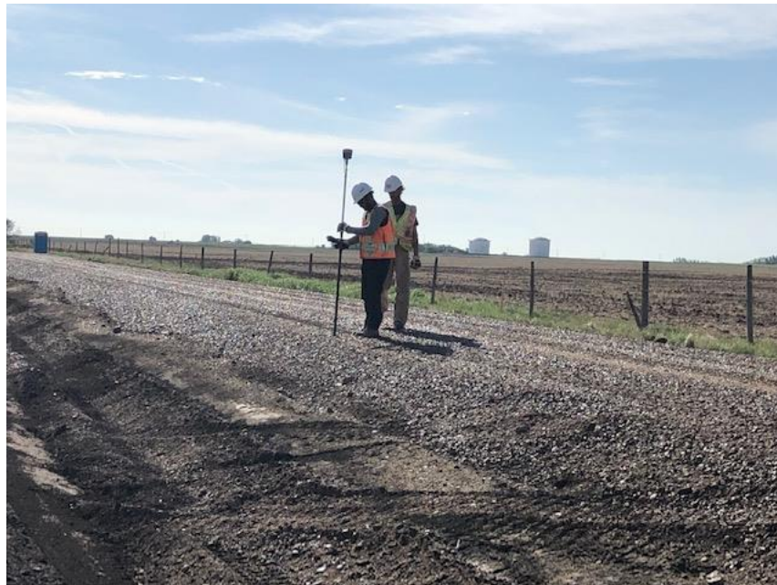
Surveyors taken measurement along the width of the road.
