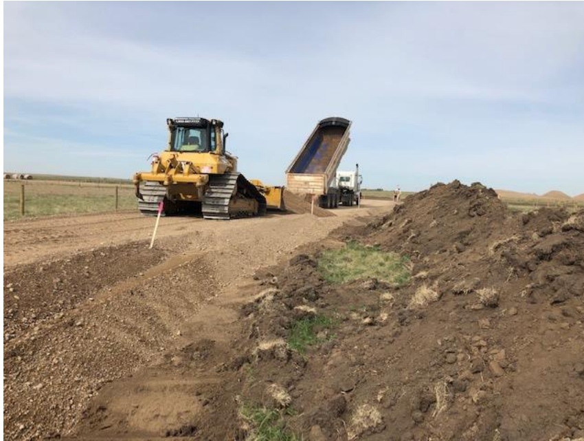
Gravel truck and Dozer spreading Pit mine gravel on access road to MLB Valve #14
