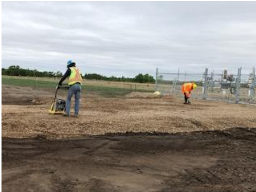
Crew manually compacting near MLB Valve #14
